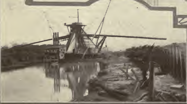
Types of French dredges used in the Atlantic entrance of the Canal as early as 1888. Those found available were rebuilt by the Americans and seven of the ladder dredges are now in use.
