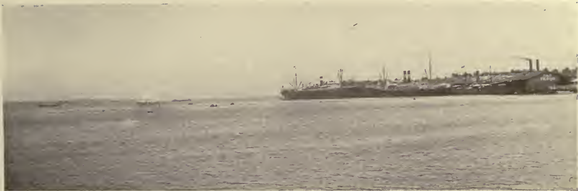
Atlantic entrance of the Canal, showing Cristobal docks.
